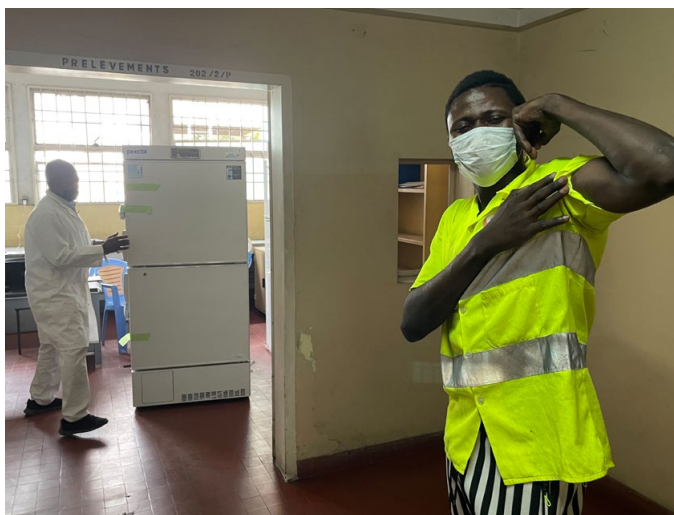
Installation of PHCbi equipment. National Institute of Biomedical Research, Democratic Republic of the Congo
